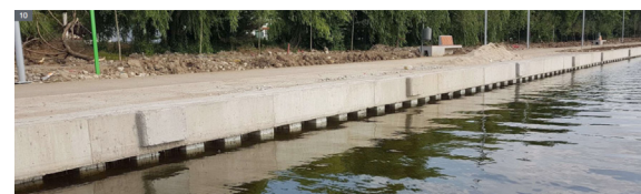
Sheet-piles quay wall – model
