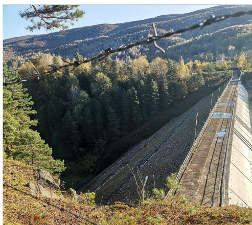
Crest of the GOZNA Dam, Caraș-Severin County
