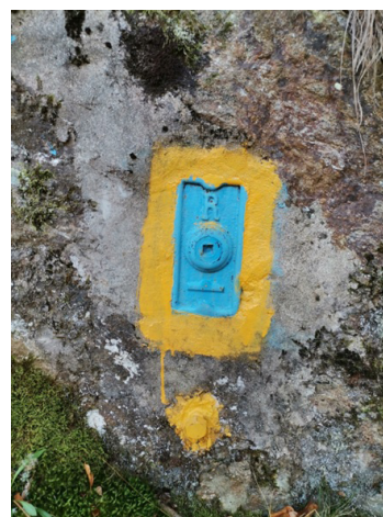
Leveling landmark, Breazova Dam, Caraș-Severin County
