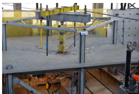
Fig. 5. Experimental test on 3D composite frame system
