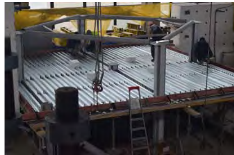
Fig. 6. Composite slab system during construction
