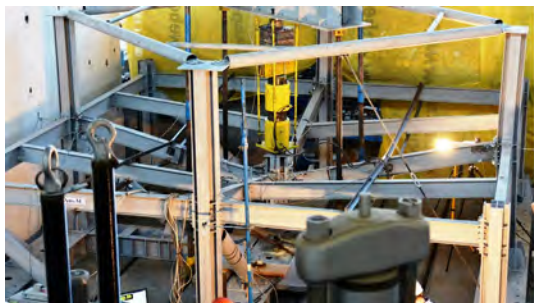
Fig. 4a. Experimental test on 3D steel frame system
