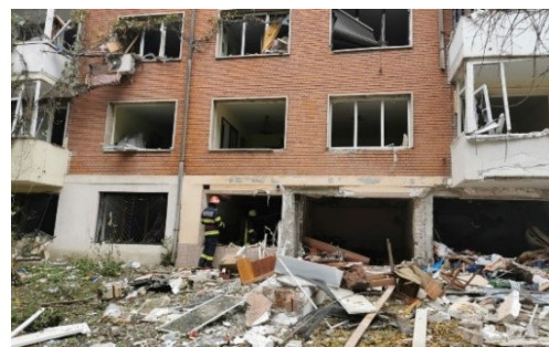
Fig.1. Gas explosion in an apartment building, Galati, 2020
