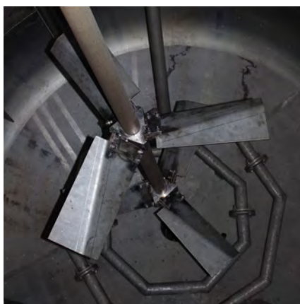
The new mixing solution installed and tested in-situ.
