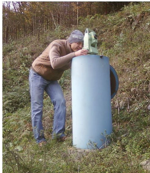
Carrying out topographical measurements for the SECU Dam, Caraș-Severin County
