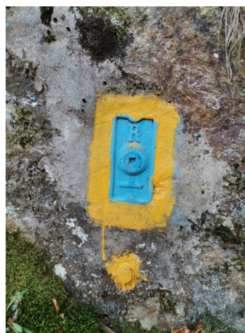
Leveling landmark, Breazova Dam, Caraș-Severin County
